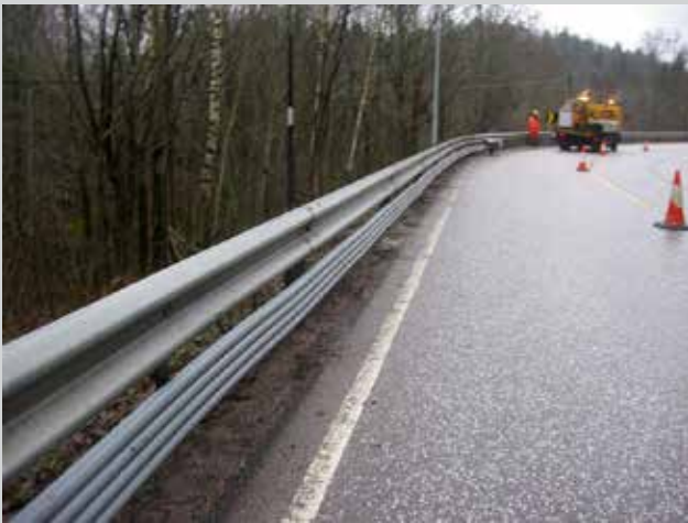
Picture 22 - Polyethylene subrails have been added to guardrails in outer curves.
