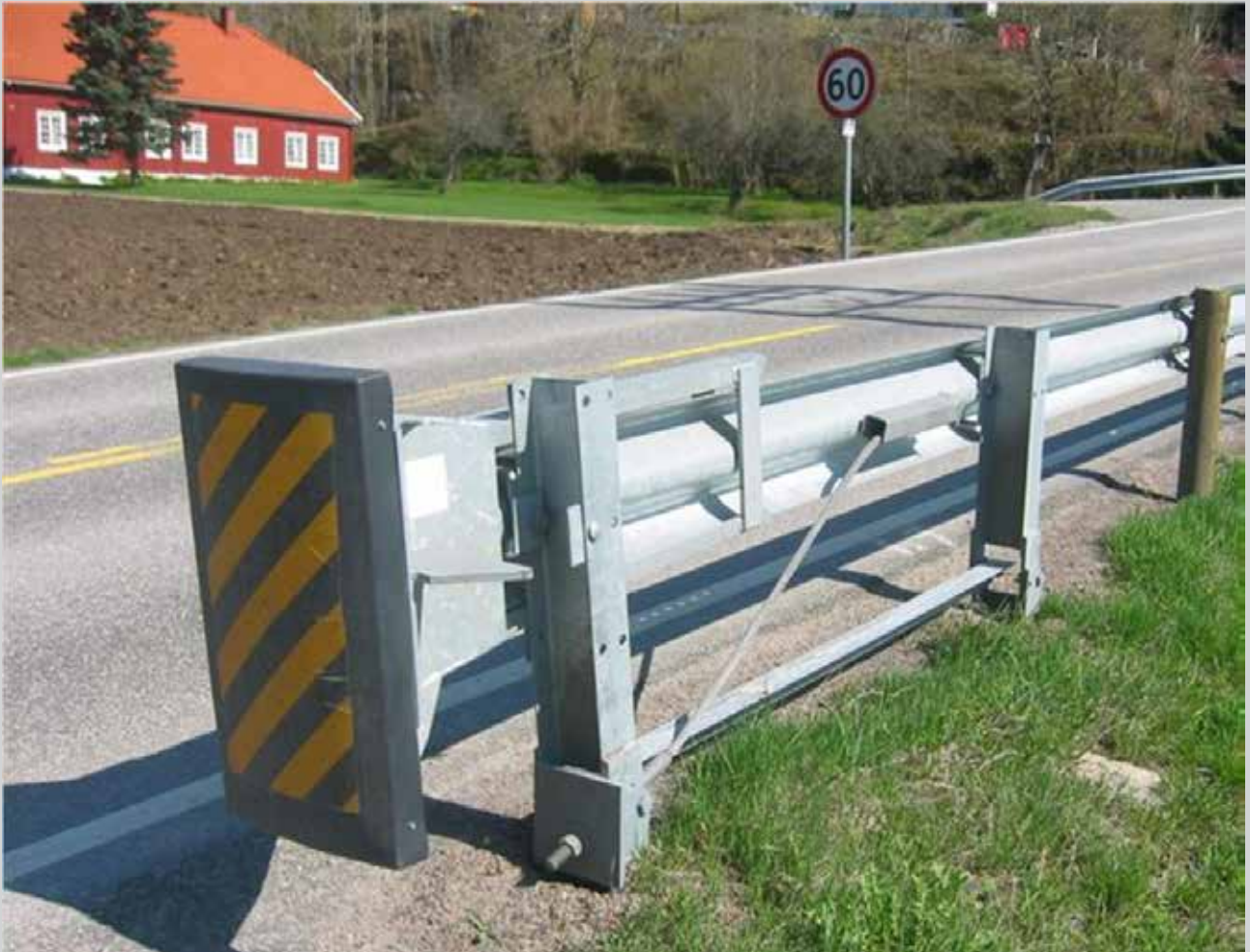
Picture 26 - Guardrail terminals present sharp edges and a low contact surface, face traffic directly and are located very close to the roadway. Fitting them with a protective cover reduce the risk of injury on impact.
