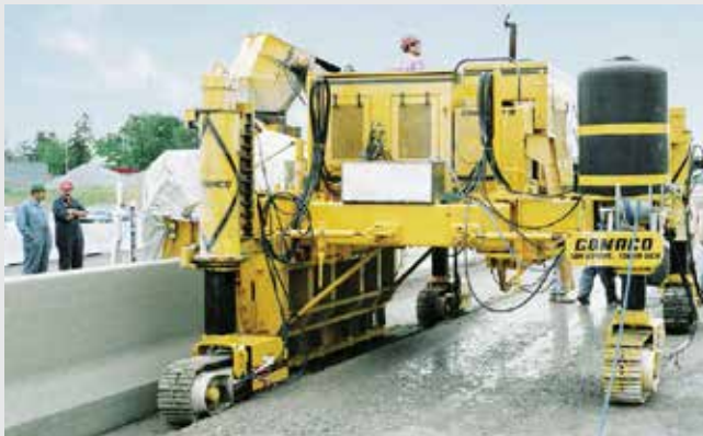
Picture 5 - slip formed concrete barrier
