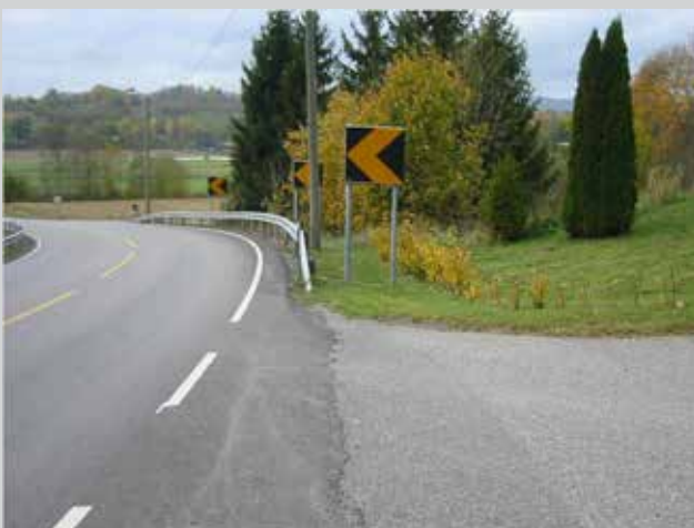
Picture 25 - Dangerous terminals have been replaced with MPS swinging away from the roadway.
