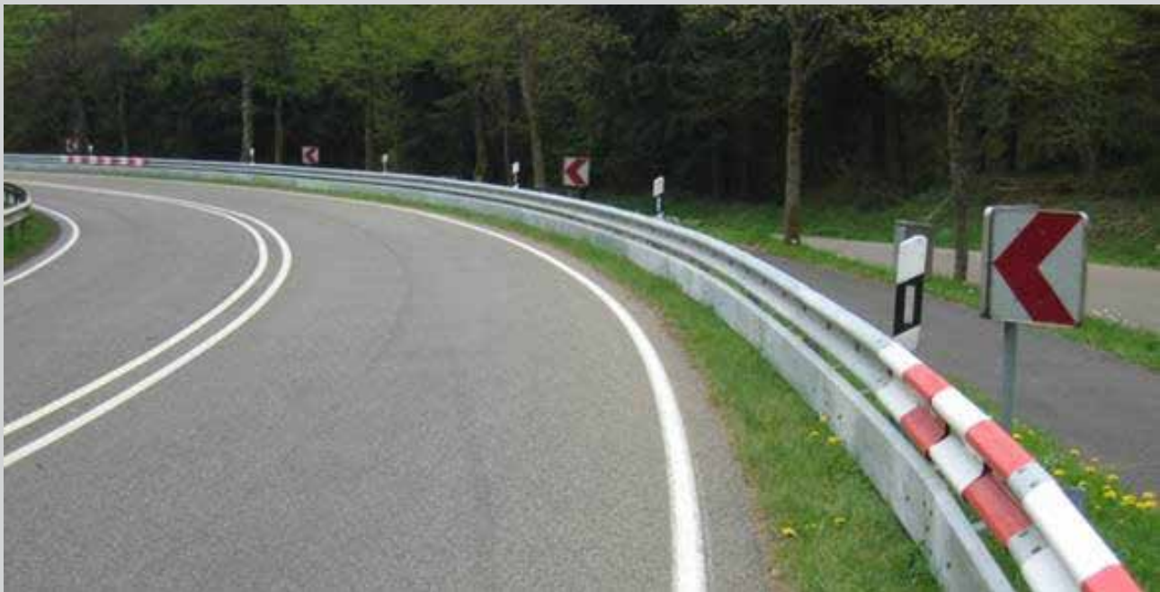
Picture 16 - Signs dispersed behind a motorcyclist protective rail
