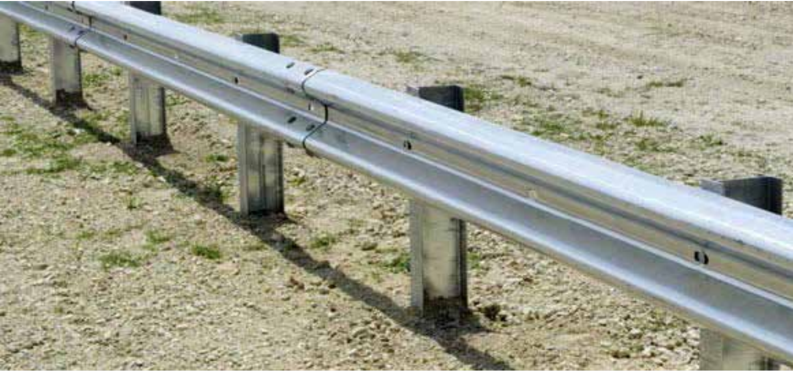
Picture 3 - normal steel guardrail
